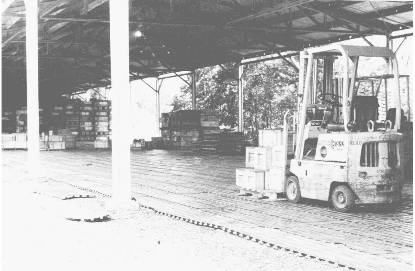
Figure 4-3. Flooring in shed area upgraded by use of steel military landing mats.
