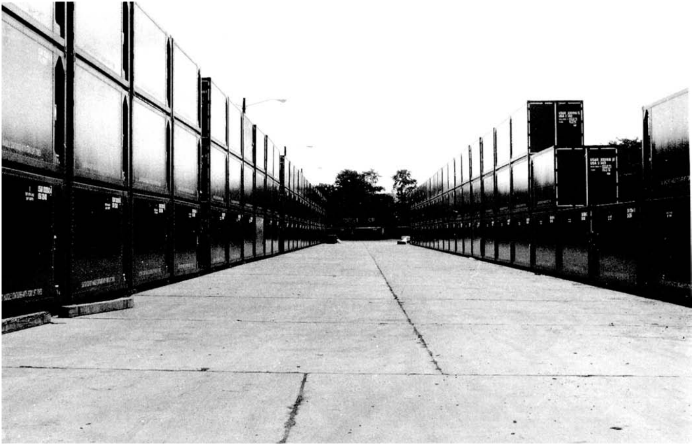
Figure 4-6. Containers stacked 3 high on concrete pavement.
