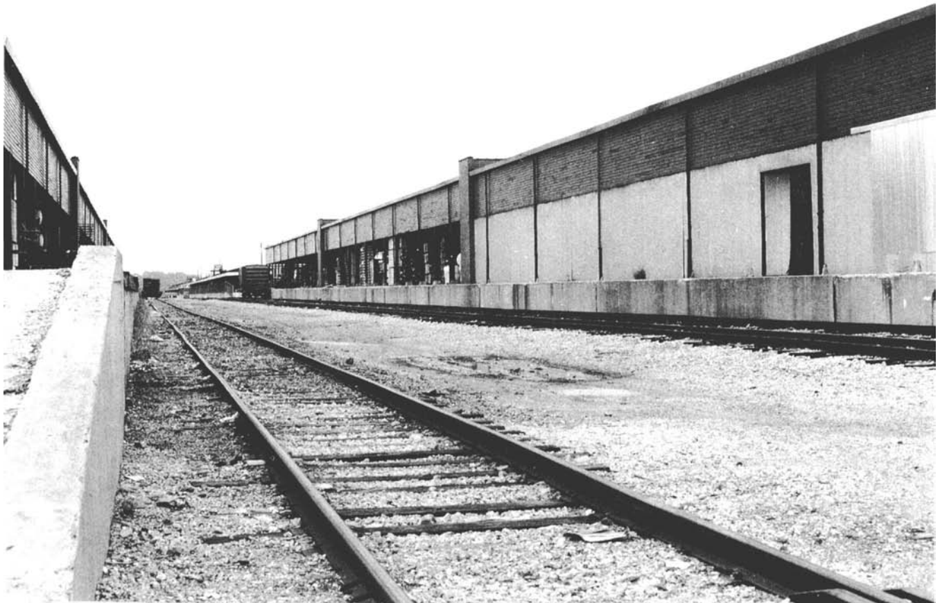
Figure 4-5. Open-sided storage shed upgraded with metal wall panels.
