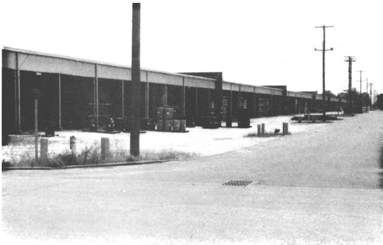
Figure 4-1. Storage shed with floor at road level.
